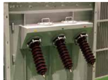
hand hole structure
