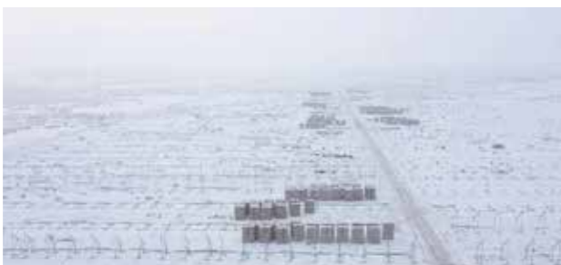
Xinjiang Lixin 37.5MW/150MWh Energy Storage Project SC(B)-2750/37kV Cast Resin Dry Type Transformer
