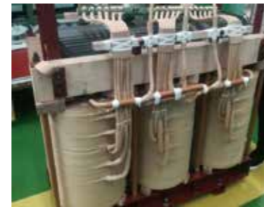
wood clamps structure
