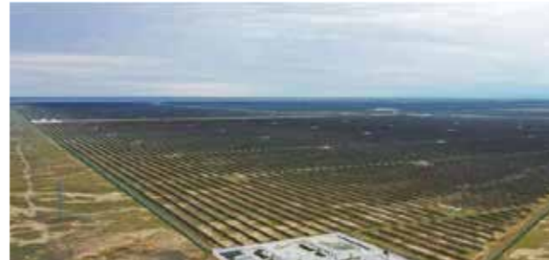
Xinjiang Mulei 125MW Energy Storage Project SC(B)-2800/37kV Cast Resin Dry Type Transformer
