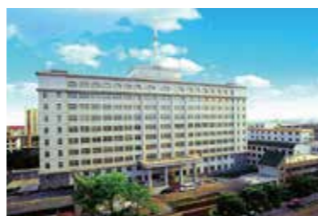
Electrical Engineering Co.,Ltd. of China Railway 12th Bureau Group
